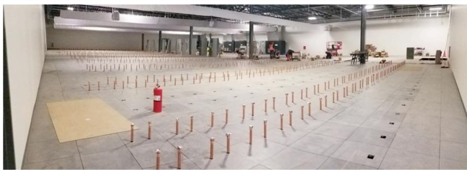
Inside Skybox data hall 2, future home of DUG’s ~40,000 KNL nodes. 5,000 1,000-litre IBCs will be brought in to fill all the tanks with coolant. (Photo provided by DUG.)
